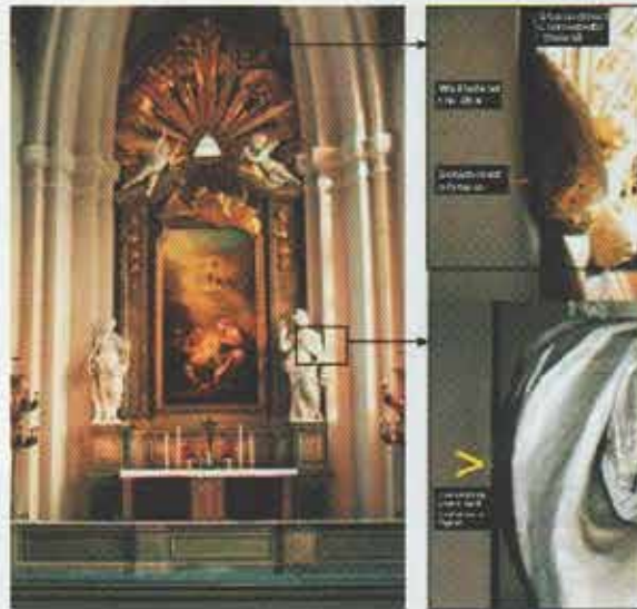
Fig. 1: Examination of the wall-integrated altar in Maria Magdalena church. Zones where the altarpieces have a direct connection to the wall. Photo: A. Henningsson
