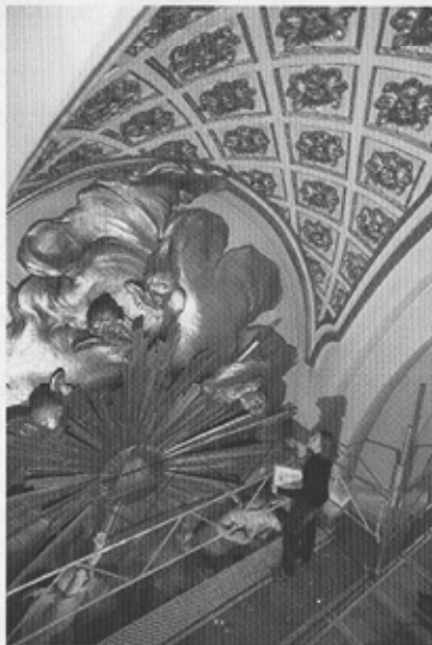
Fig. 6: Condition survey by mapping of the stucco altar in Maria Magdalena church. Photo: H. Ekestang
