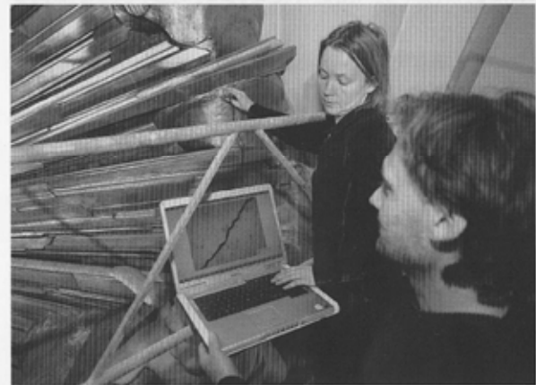
Fig. 5: Measuring crack width in stucco using microscope. Photo: H. Ekestang
